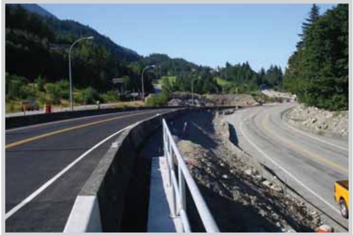
New northbound lanes at Furry Creek include a new bridge
