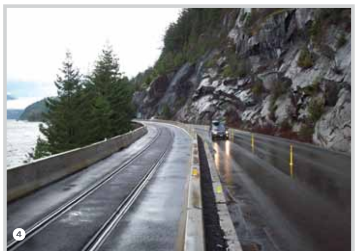
4 The completed temporary third-lane at Porteau Cove,, north of Horseshoe Bay.
