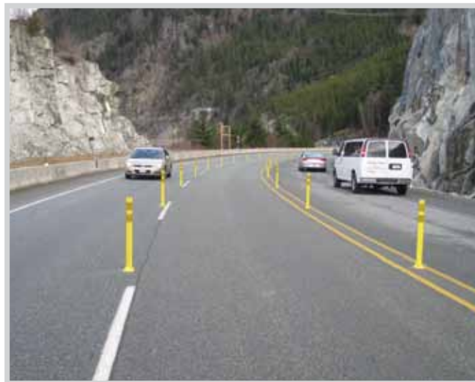
Between Squamish and Whistler, three-lane sections will operate in a two-lane north, one-lane south configuration marked by temporary yellow lane markers.
