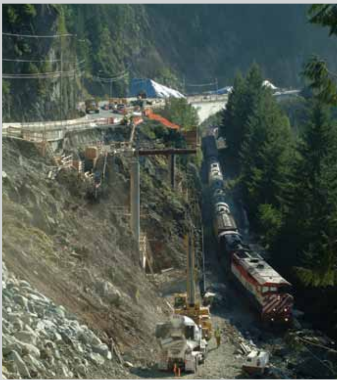
BEFORE: Highway construction just south of Strachan Road.
