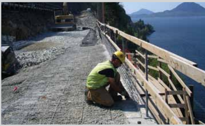
The team made extensive use of downslope construction, building nearly 60,000 square metres of mechanically stabilized earth (MSE) walls. This work, along with the 'half bridges', eliminated the need for major upslope blasting and extensive road closures.
