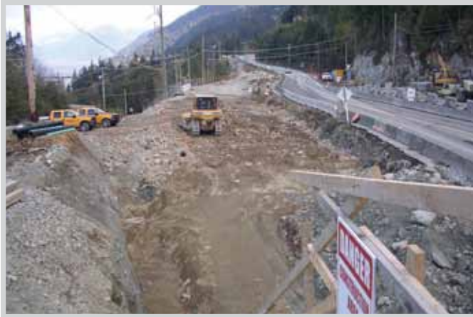
BEFORE: View of Lions Bay from Kelvin Grove overpass.
