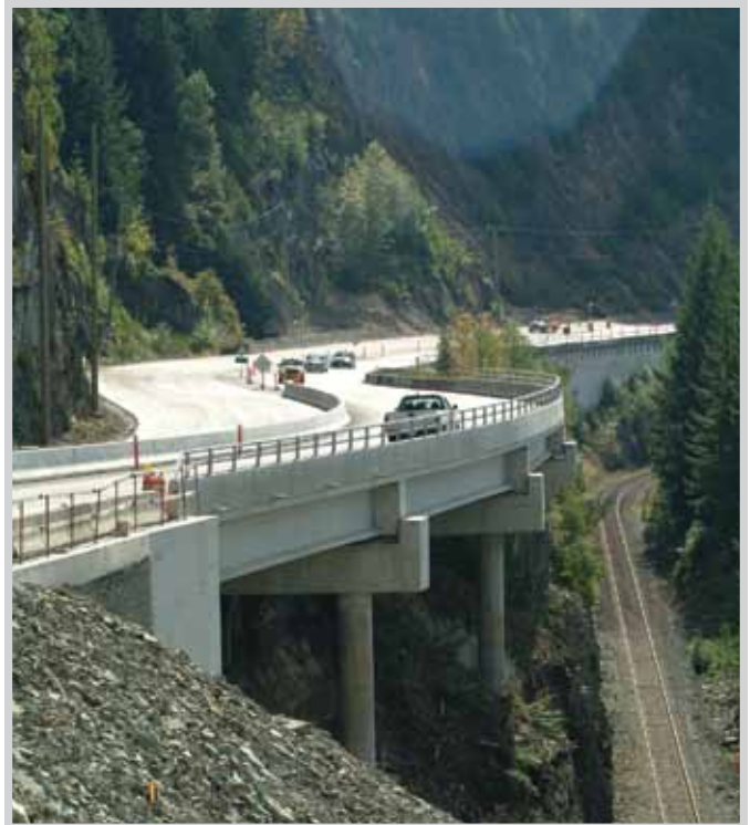
AFTER: Same location post-construction. This view is an example of downslope construction minimizing the need for upslope blasting and extensive road closures required to clear blasts. Designers and engineers made extensive use of mechanically stabilized earth (MSE) walls and in this photo, "half bridges" to extend the highway and the two new lanes.
