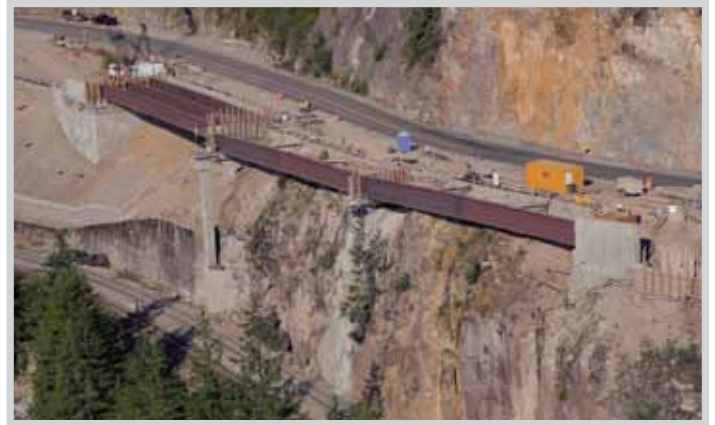
The team made extensive use of downslope construction, building nearly 60,000 square metres of mechanically stabilized earth (MSE) walls. This work, along with the 'half bridges', eliminated the need for major upslope blasting and extensive road closures.
