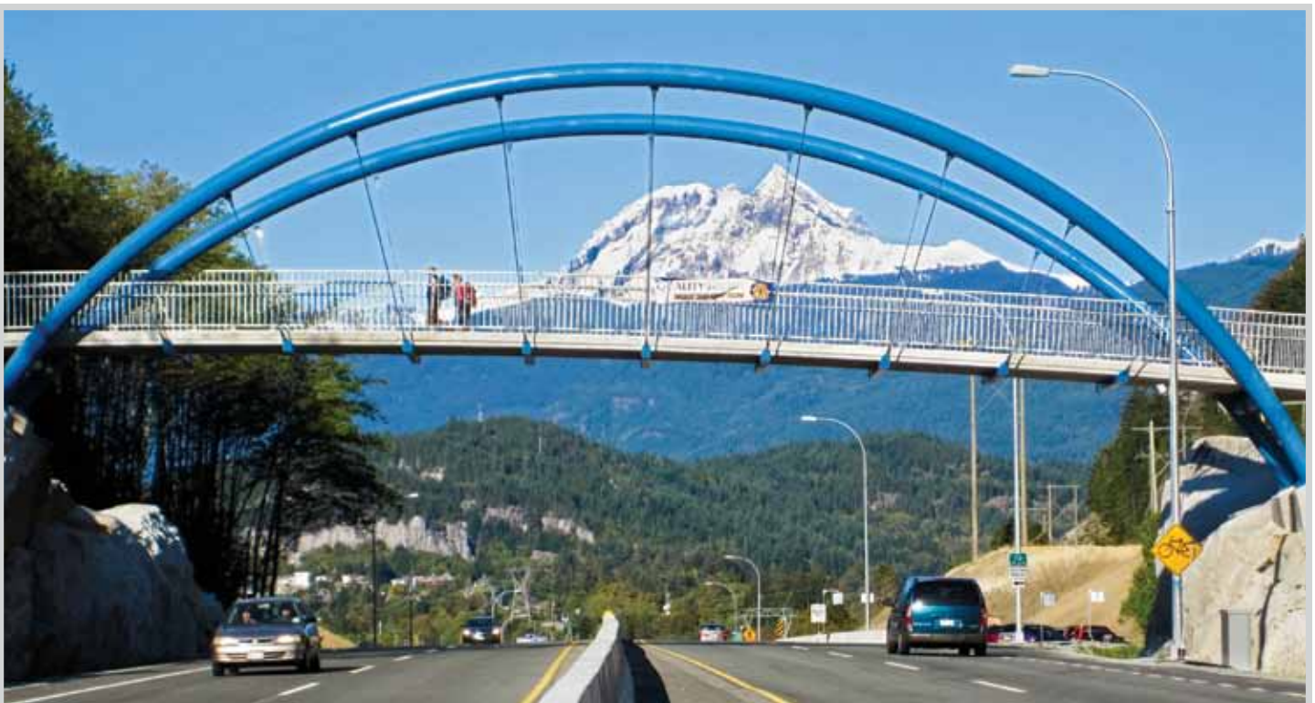
Improvements were made to community recreation assets along the corridor. Shown here, a new pedestrian overpass at the Stawamus Chief Provincial Park, where improved access and enlarged parking facilities will improve safety for climbers and hikers.
