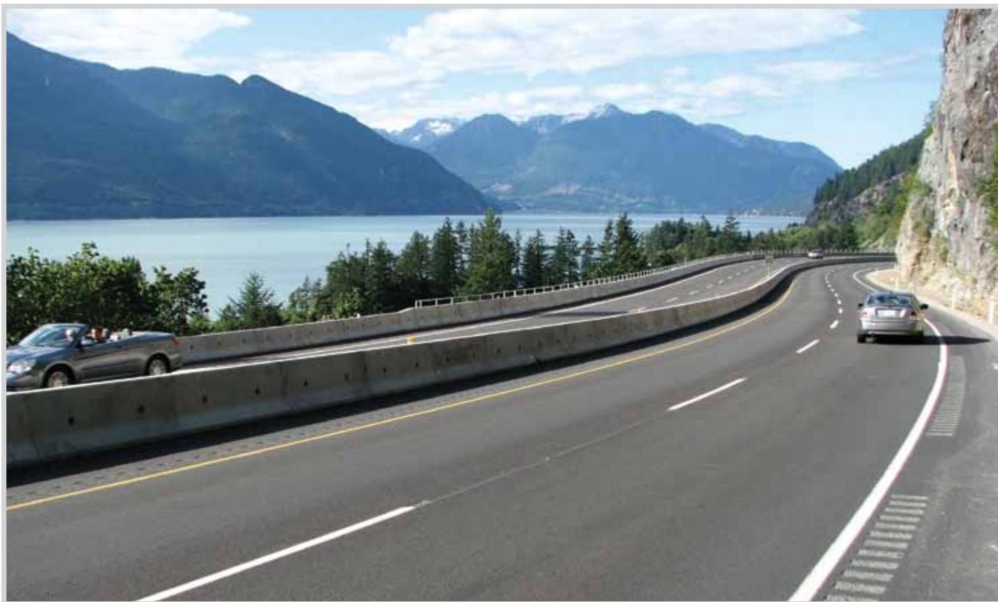
Increased lanes, centre median barrier, rumble strips and improved highway markings are shown in this section of new highway north of Lions Bay. Eighty kilometres of new passing lanes have been added due to the Sea-to-Sky Highway Improvement Project.
