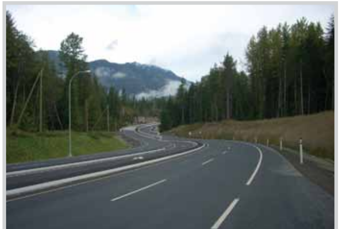
AFTER: Garibaldi Park entrance to Cheakamus Bridge post-construction as multi-laned highway with a protected T intersection, raised medians and median barriers, 1.5-metre shoulders, smoother curves and improved sightlines.
